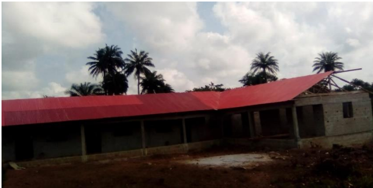
The building with the roof nearing completion:
